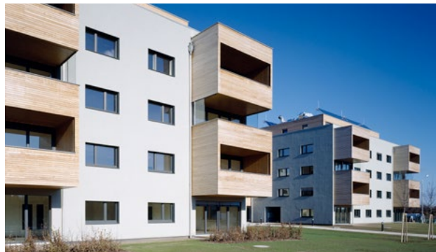
Timber passive house on Mühlweg, 1210 Vienna, photo: Bruno Klomfar
