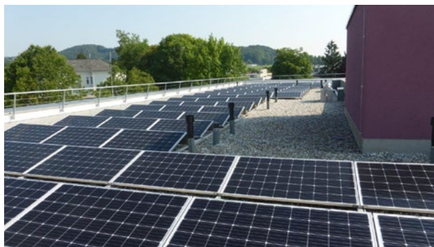
Itzling care home, block 4, photo: City of Salzburg, Georg Pirchner
