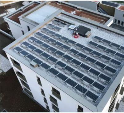
Photovoltaic system with a total output of 140 kWp. The electricity generated during the daytime can be distributed between all residents by a dynamic calculation method and used immediately. Photo: SIR
